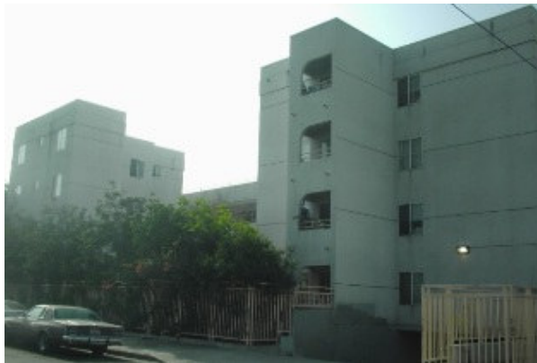
Central Avenue Villa, before rehab
